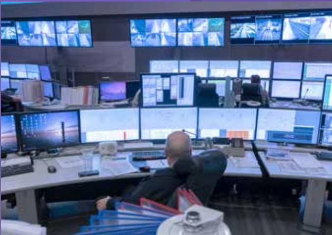
Mipro's ATS in the Herttoniemi control centre in Helsinki manages the metro traffic in the Finnish capital area.
